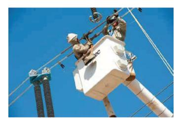
dures was the ability to adapt to job irregularities. A necessary adaptation that occurred early in the project was related to the bundled conductor, which sat in a vertical configuration rather than the tradition horizontal configuration. To most efficiently tackle this issue the team needed to adapt both the equipment and the procedures. This first test proved to be a calling card for the entire project as procedures were continually updated to make the project safer and more efficient.
