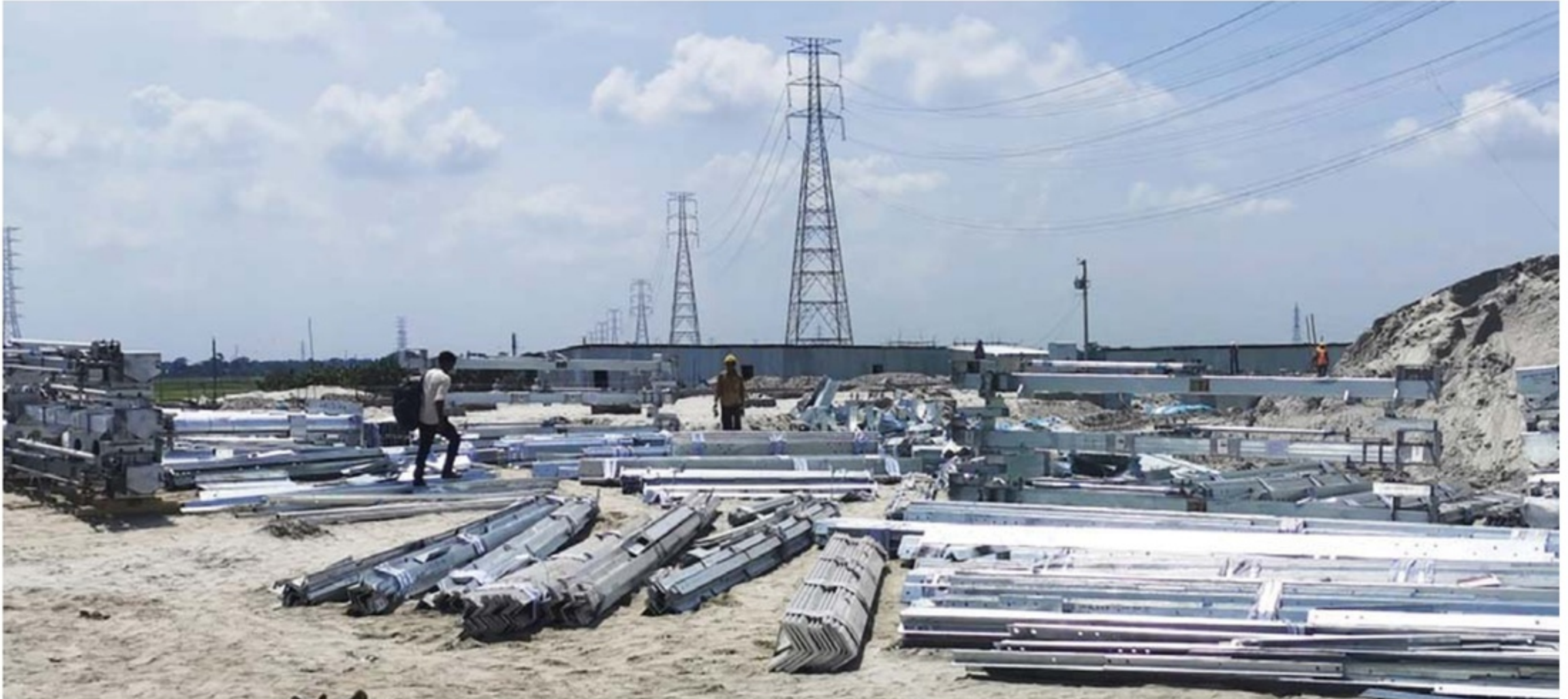
View of 400-kV tower from Gopalganj substation.
