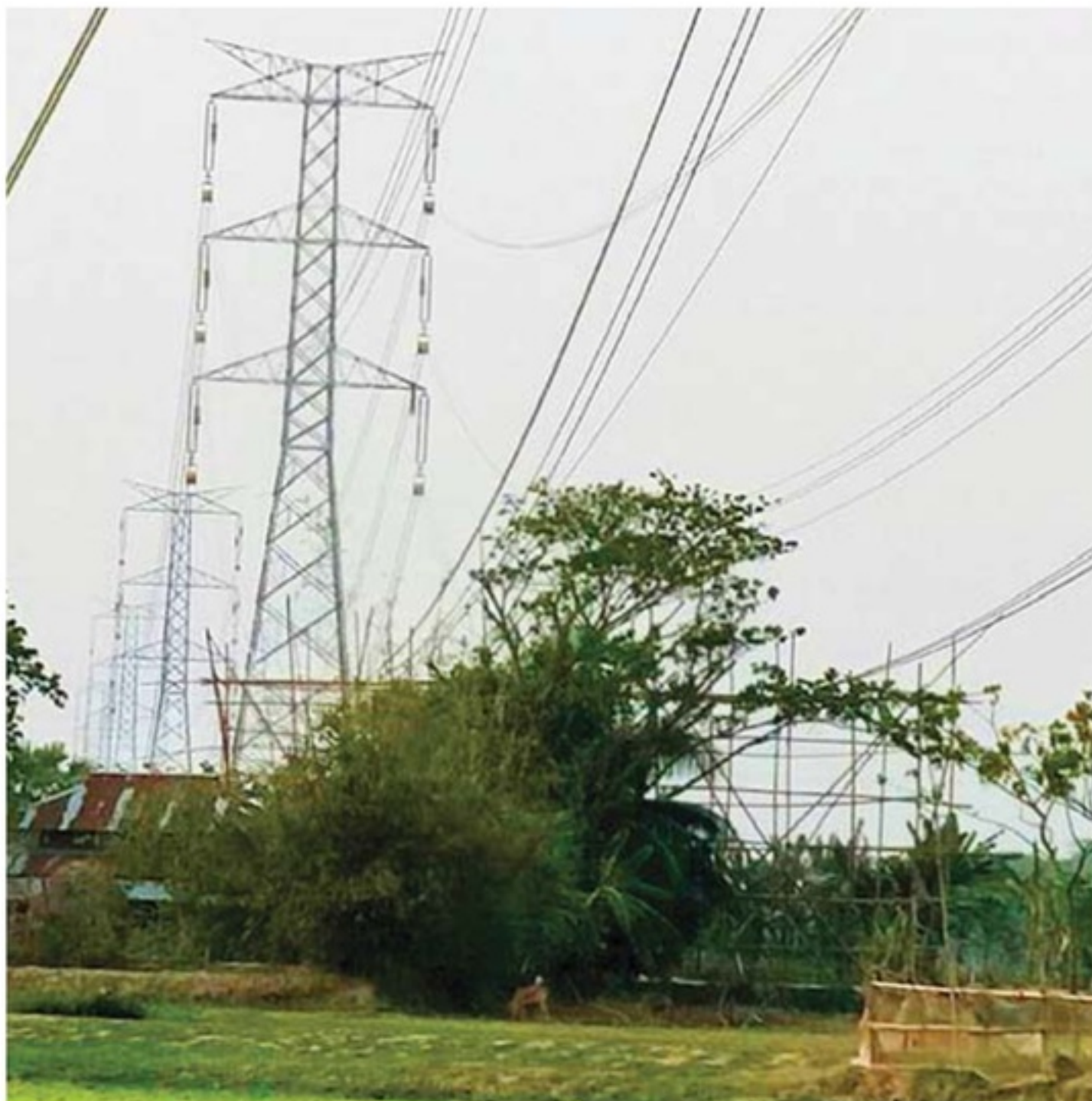
Large 400-kV terminal tower in Payra.
