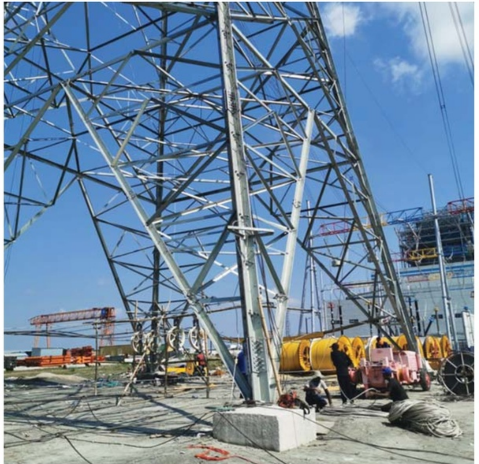
Conductor stringing works near Gopalganj substation.
