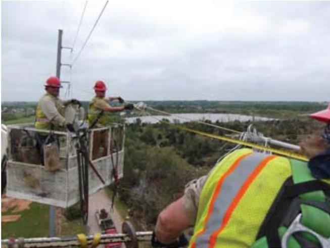
**Fig. 5 :** OG&E linemen preparing to install 4 meters of ACCC Conductor to repair tornado damage
